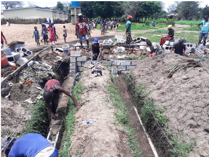
Figuur 8: Start fundering school fase 2
